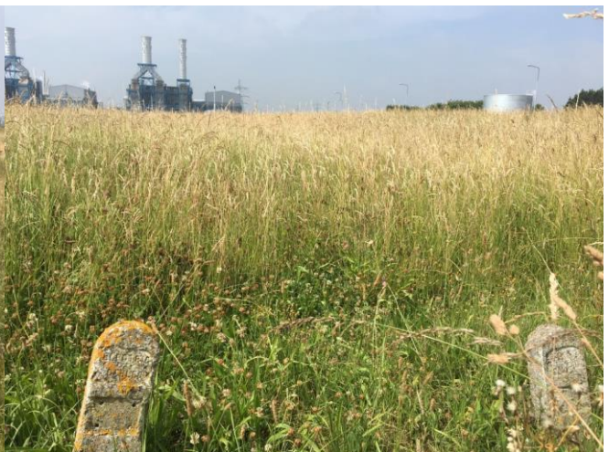
(4) Ground markers (buried pipework)
