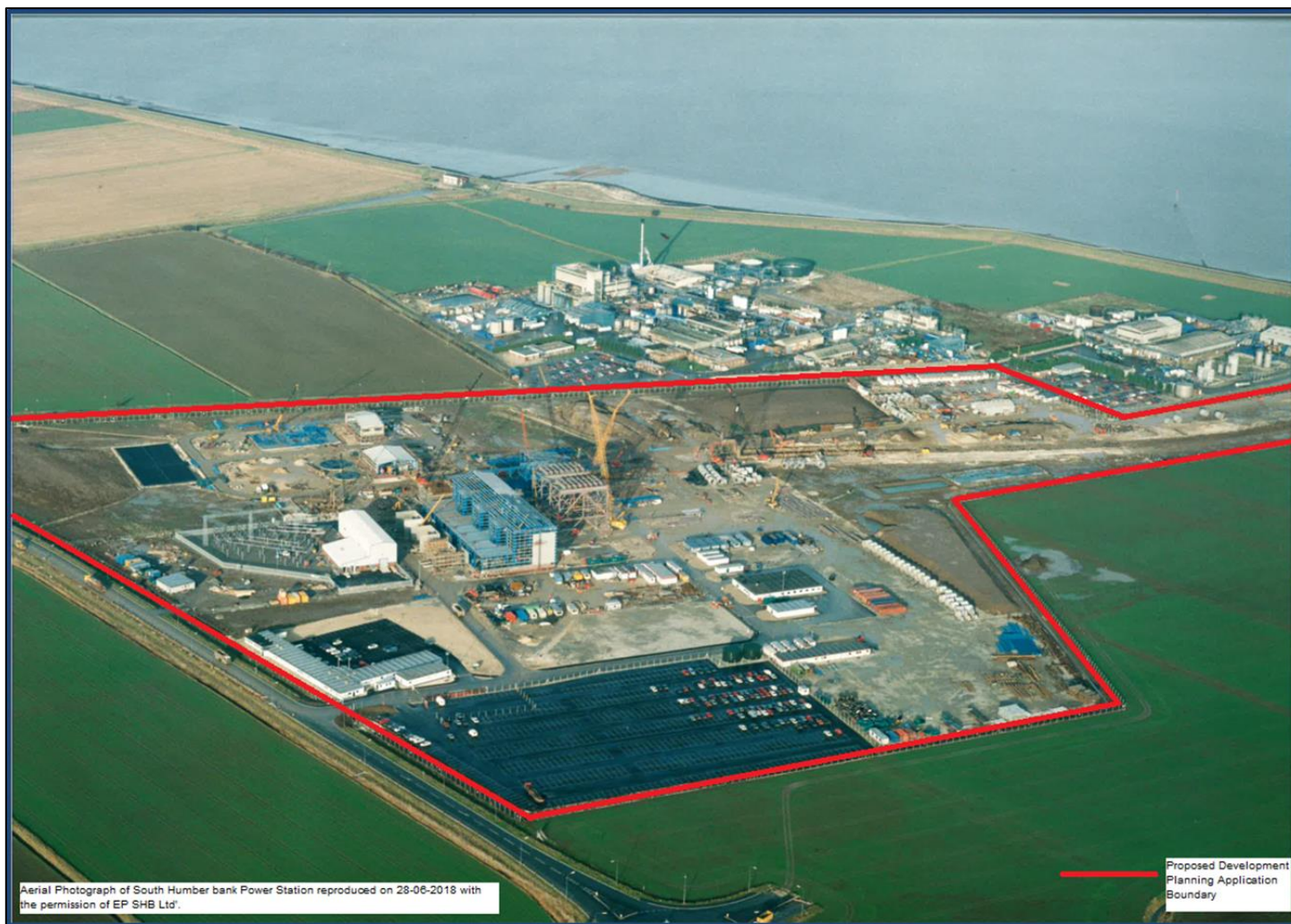
Plate 4 Aerial Photograph showing areas of the Site disturbed during the construction of South Humber Bank Power Station.
